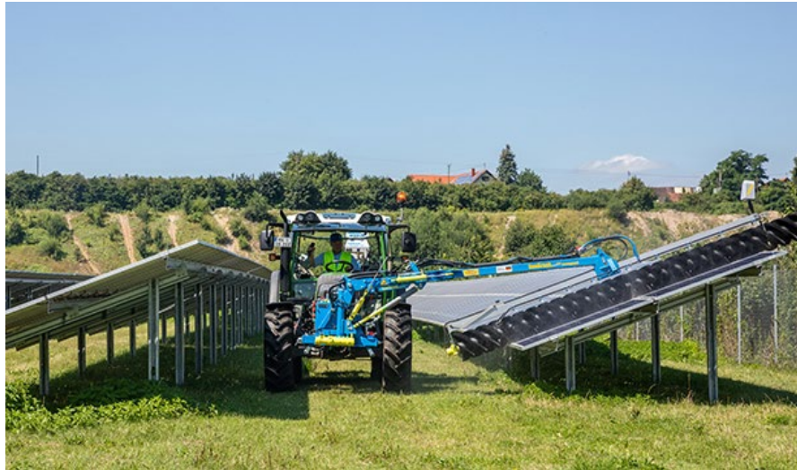
Figure 12- Solar PV panel Cleaning Method
