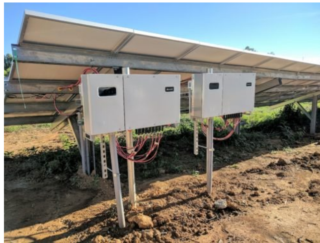
Figure 2- String Inverters
